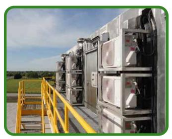
Along the exterior side of these Off-Shore Living Quarters, designers provided wide walkways, safety railing and room for caged Bebco Split System Condenser Units, stacked three-high to minimize space consumption. Each Bebco Split System Condenser Unit is then separately connected to a corresponding Evaporator Unit, deep within the structure, which provide the critical heating and cooling required to keep billeted crew members comfortable!
