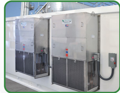
Model VAC Units provide N+1 cooling and heating for this expansive Control Room located in a Gulf Coast Refinery
