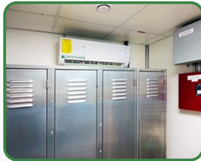
This Crew Quarters Locker Room benefits from the remote controlled cooling force of a Bebco Model SAC Split System Evaporator Unit
